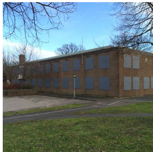
The boarded-up Police Station building
