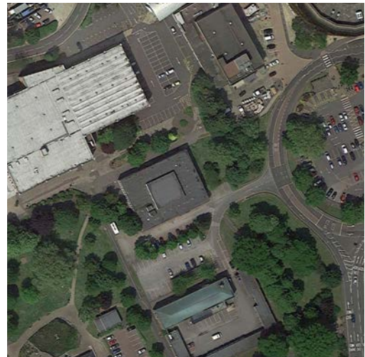
Existing site area
