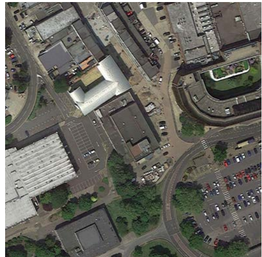
Existing site area
