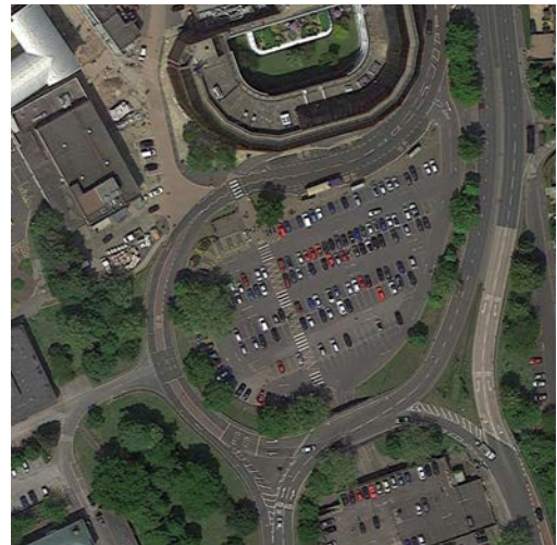
Existing site area
