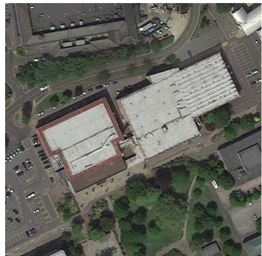
Existing site area
