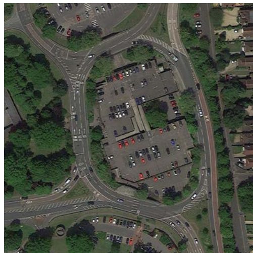
Existing site area
