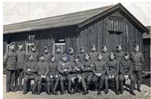
The Pinehurst Barracks (Elles Barracks from 1934) which was demolished in 1970s. The Sergeants Mess is used as the Farnborough Community Centre
